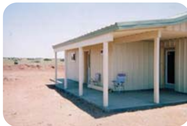
Covered Exterior Walkway ©Joel Kapp
