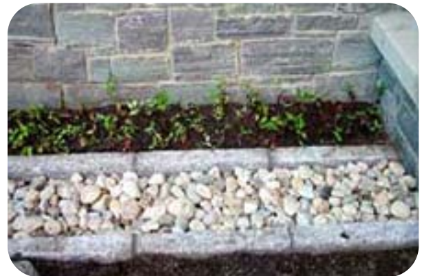
French Drain ©JES Construction, Inc.
