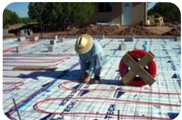
Laying Radiant Heating Pipes ©Melinda Honn
